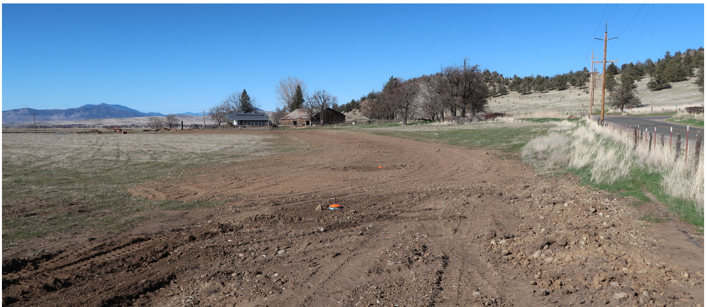
Figure 2. New mainline system
