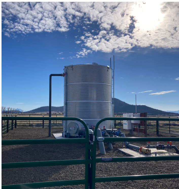
Figure 3. Main tank of new pressurized stockwater system which will allow for more efficient year-round livestock watering and will remove cattle from the stream
